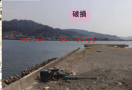
⑧堤防破損
