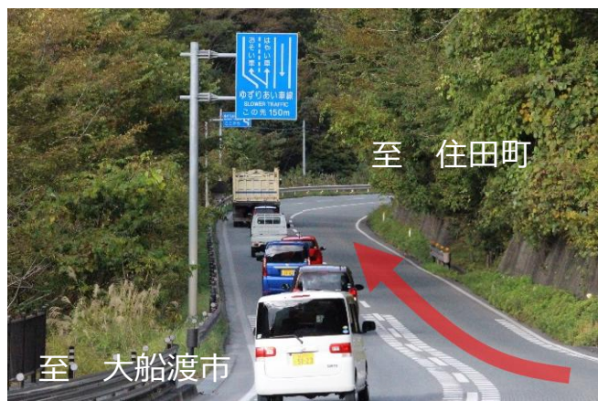
②急勾配 (縦断勾配8.4%)
