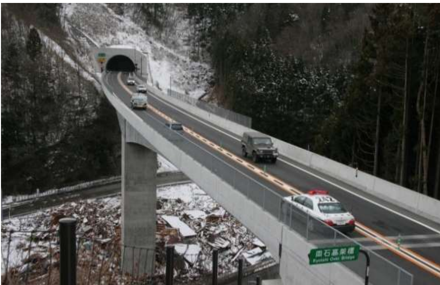
The Kamaishi-Yamada Road opened on March 5, 2011
