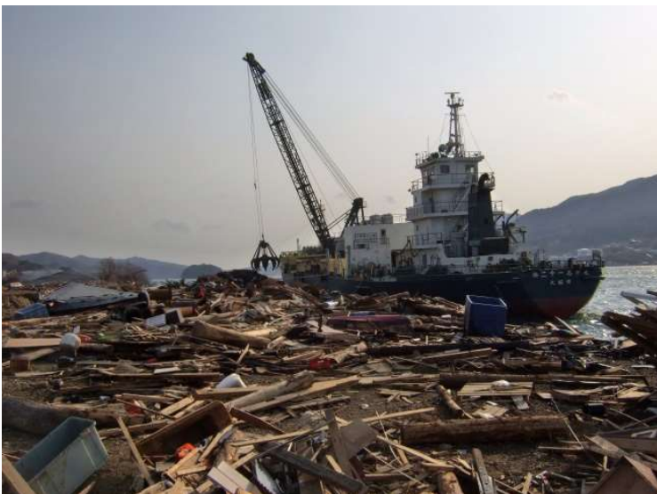
Sea Clearing Work at Ofunato Port
