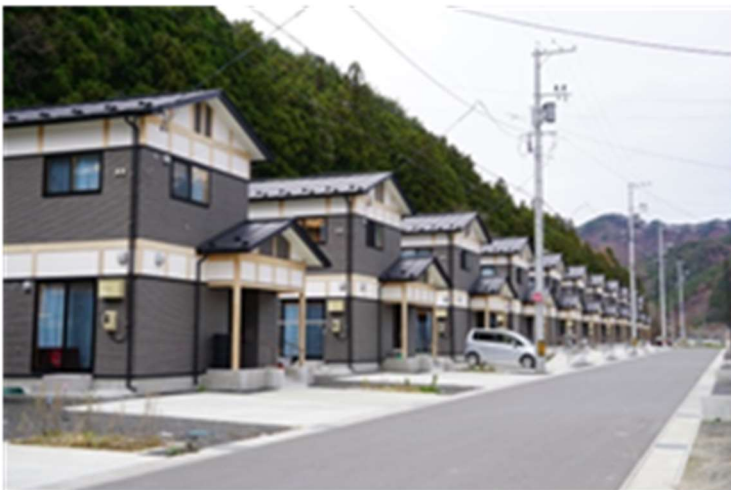
Terano (Phase 1) Disaster public housing (wooden, detached) in Otsuchi Town, completed in September 2015.
