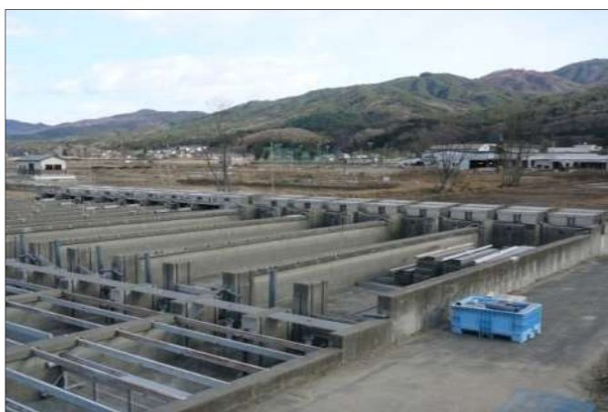
Tsugaruishi Hatchery, Miyako City after emergency restoration
