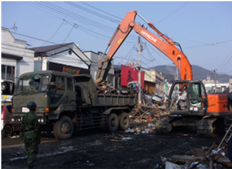
Road Clearing Work in Kamaishi City (March 13th, 2011)
