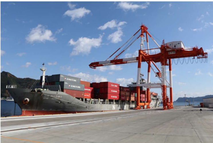
Container loading and unloading by gantry crane (November 17, 2017) Kamaishi Port
