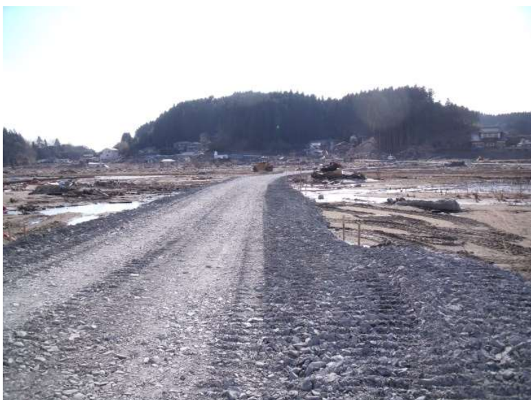
Ofunato Hirota Rikuzentakata Line (Rikuzentakata City)
