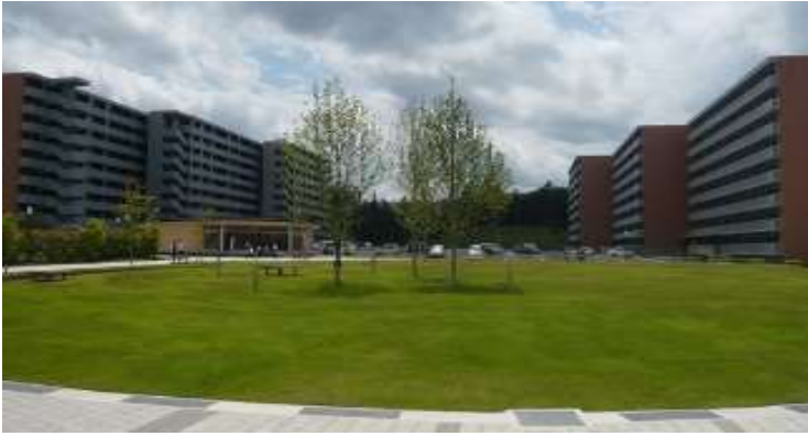
Tochigasawa Disaster public housing in Rikuzentakata City completed in June 2016 (301 units, 9 floors, the largest in the prefecture)
