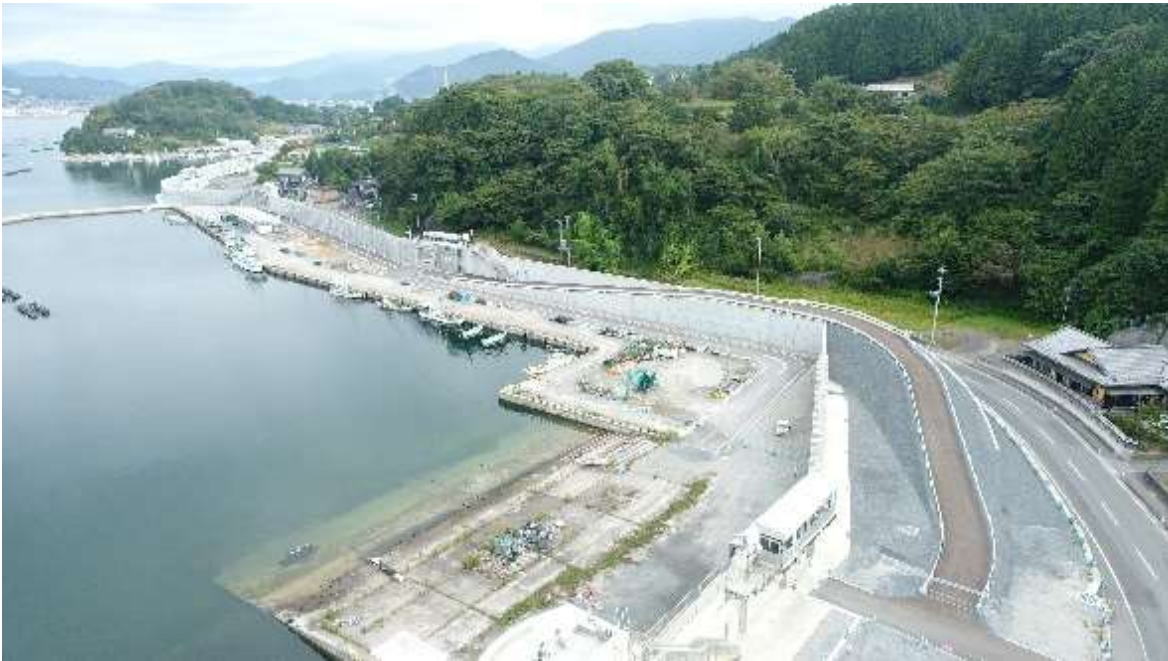
Ofunato Port Coastal Shimizu Area Seawall completed in the 2022 fiscal year (Ofunato City)
