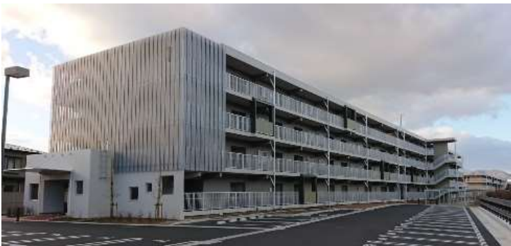
Minami Aoyama Apartments (for inland evacuees, 99 units, some 4 stories) in Morioka, completed in December 2020.
