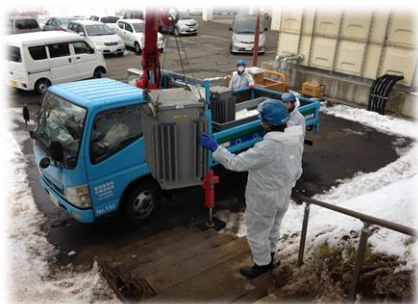
PCB廃棄物の搬出風景
