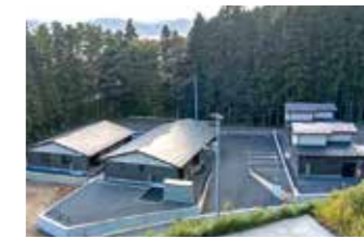
Public housing in the Ando area of Otsuchi (completed in December, 2018)
