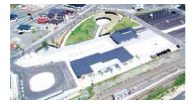
The completed "Kamaishi Memorial Park", "Tsunami Memorial Hall" and "Unosato Visitor Center" (Opened for use in March, 2019)
