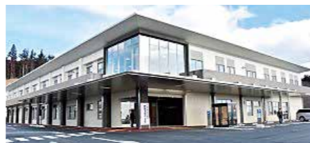
Takata Prefectural Hospital
