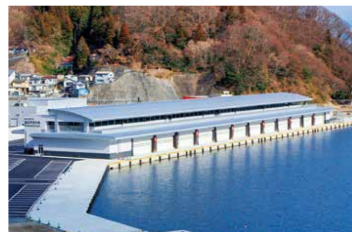
Kamaishi City Fish Market: Completion of a highly sanitary fish market (Completed in May, 2017)
