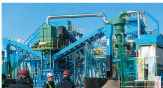
Disaster waste treatment demolition and sorting line established in Miyako
