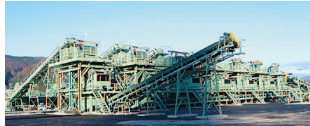
Salt removal facility
