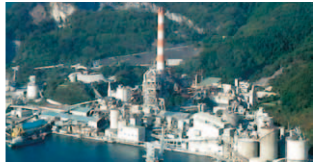
Taiheiyo Cement Corporation's Ofunato factory
