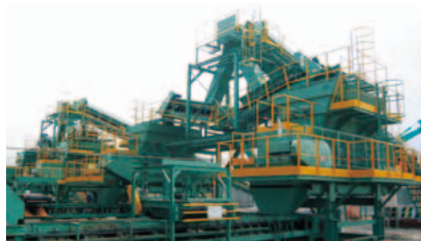
Soil classification treatment facilities at Rikuzentakata (Joint venture with Rematec. Ltd.)
