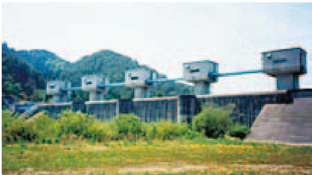
Floodgates that helped to mitigate damage from the tsunami in Fudai
