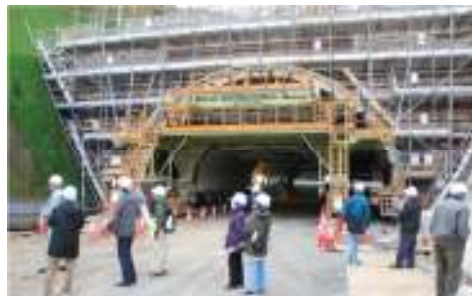
The Ube Tunnel construction site
