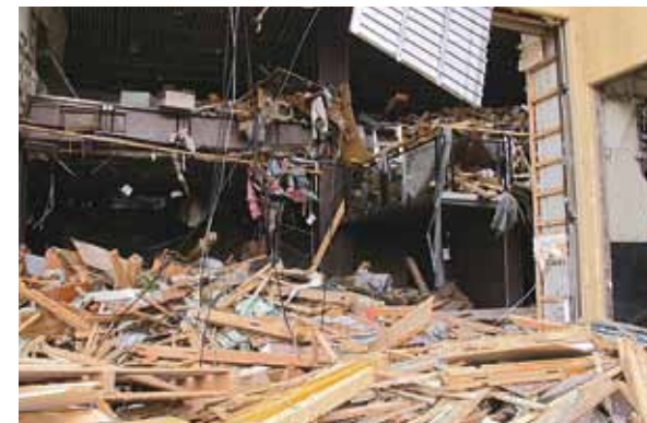
The interior of the damaged Rikuzentakata City Museum
