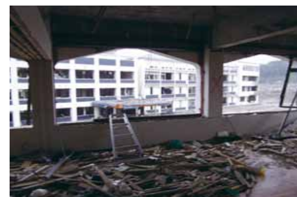
The damaged office of Rikuzentakata City Board of Education
