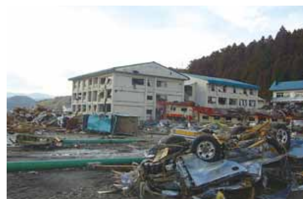
The damaged school building of Takata High School
