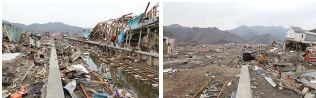
Otsuchi Station destroyed by the tsunami and fire
