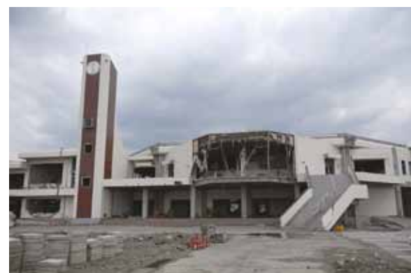
Completely destroyed Rikuzentakata Civic Gym
