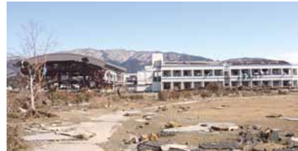
Completely destroyed Prefectural Takata-Pine-Covered-Shore Activity Center
