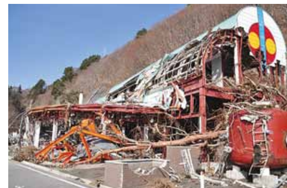
Completely destroyed Kuji Underground Aquarium
