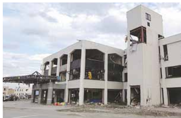
Completely destroyed Rikuzentakata Civic Center
