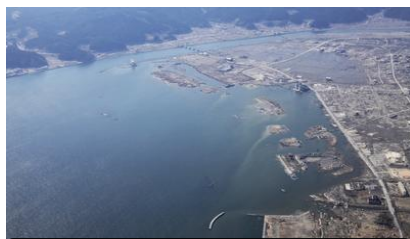
Rikuzen Takata City, Takata Pine Beach (After the Disaster) March 29, 2011
