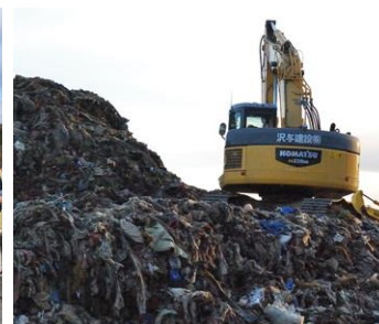
Waste processing at the Miyako facility
