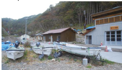
Building construction on Banyagun completed
