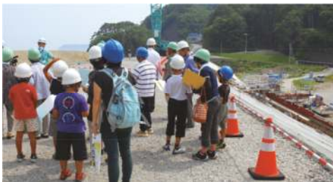
The construction site in Aketo coast (Tanohata)
