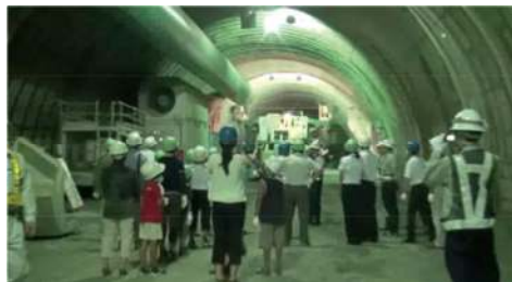
The construction site in Settai Tunnel 1
