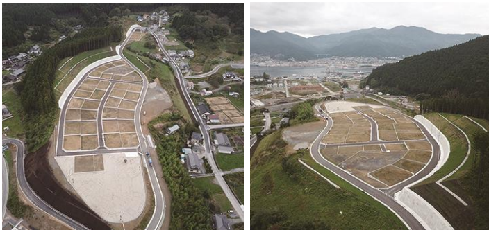
The completed land development work at Morikko/Horikawahara (Photo: Ofunato City)
