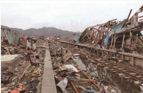
The devastated JR Otsuchi Station (Photo: Otsuchi Town)
