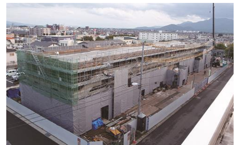
Ongoing construction at Bingo Daiichi Apartment
