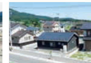
Residential area relocation in Wakinosawa, Rikuzentakata City (Completed in October 2015)
