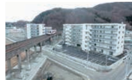
Public housing for survivors in Matsubara, Kamaishi City (Completed in March 2017)
