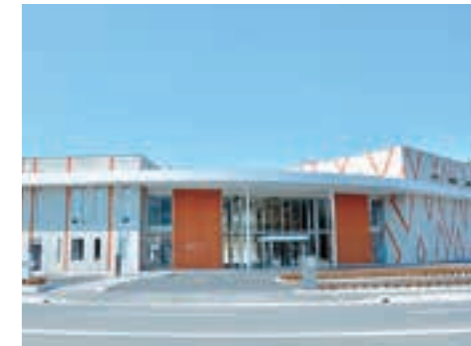
Rikuzentakata Community Hall (March 2015)
