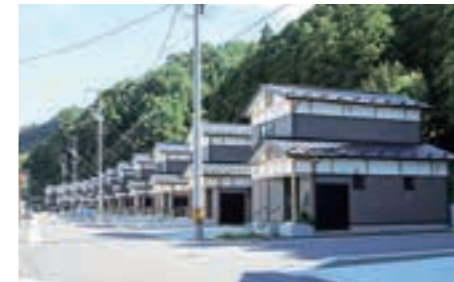
Public housing for survivors in the Terano district of Otsuchi Town (Completed in July 2016)
