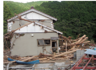
The damage by debris flow
