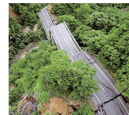
The Iwate-Miyagi Nairiku Earthquake in 2008
